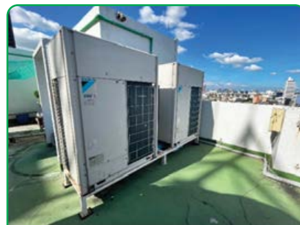
VRV air conditioning system
